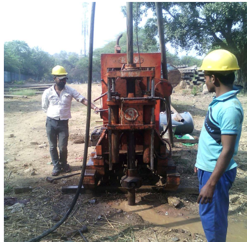
Fig. 2. Borehole Drilling in progress.
